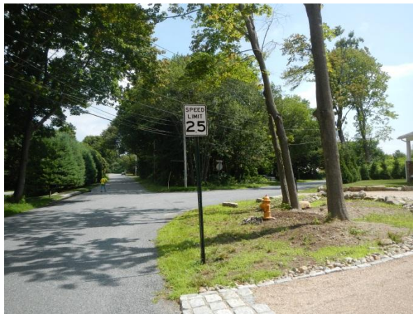
Photo 20 - Looking Northeast along Strathmore Road at Wanda Street (8-4-14)
